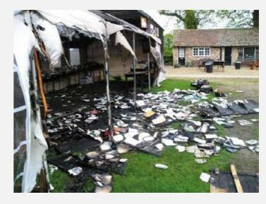
The fire has totally destroyed several sidewalls as the fire was allowed to spread by the highly flammable sidewalls of the competitor's marquee.
