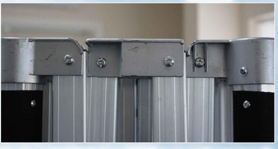
Cast metal joints which are not covered and will be prone to rubbing and damaging the canopy
