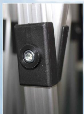
Piece of plastic around the trusses that does nothing to prevent wear and tear, and is just cosmetic. The plastic is abrasive and has sharp edges. No caps on the trusses.
